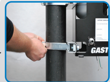
Secure lower pipe clamp
