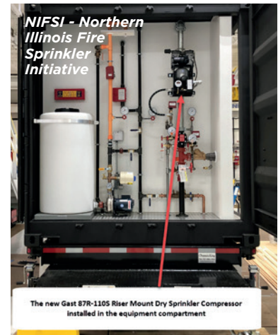
87R-110S compressor also shown in NIFSI burn trailer recently completed in 2020
