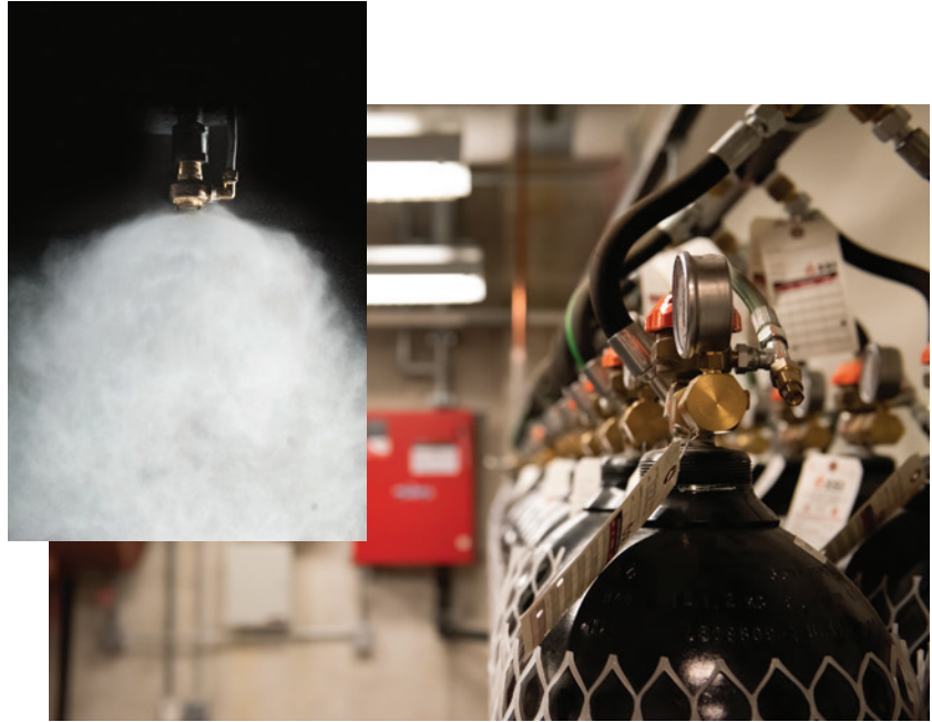
The Victaulic Vortex™ hybrid fire extinguishing system mixes nitrogen with atomized water particles, attacking the oxygen and heat legs of the basic fire triangle to suppress and extinguish.
