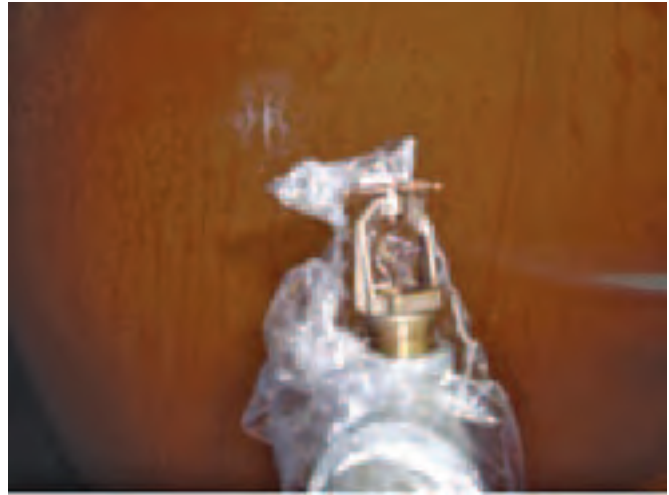
Figure 8 - Plastic bags can shrink onto sprinkler frame rather than burn away when exposed to heat and flame
