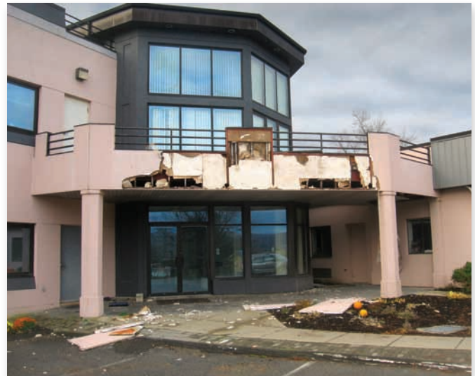
NFSA headquarters damaged by Hurricane Sandy
