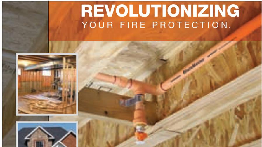
BlazeMaster® Fire Sprinkler Systems – made from The Lubrizol Corporation's superior CPVC compounds – are the first and only non-metallic systems to pass UL testing for use with exposed composite wood joist systems in unfinished areas of basements. This patent-pending application technology is transforming fire protection, proving BlazeMaster Fire Sprinkler Systems to be the innovation leader.
