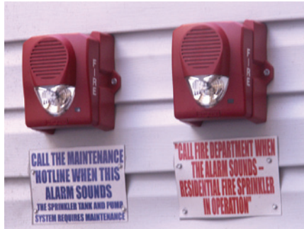
Fire and trouble alarms on Pump Tank Module
