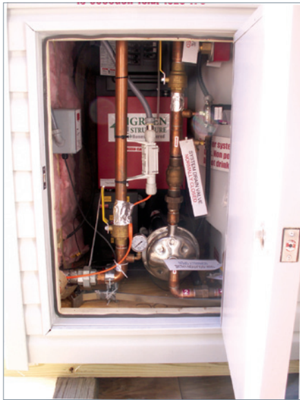
Closeup of P&T controls
