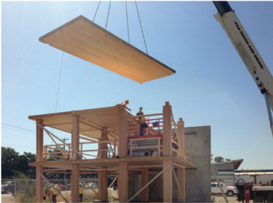
July 2015 erection of mass wood structural mockup
