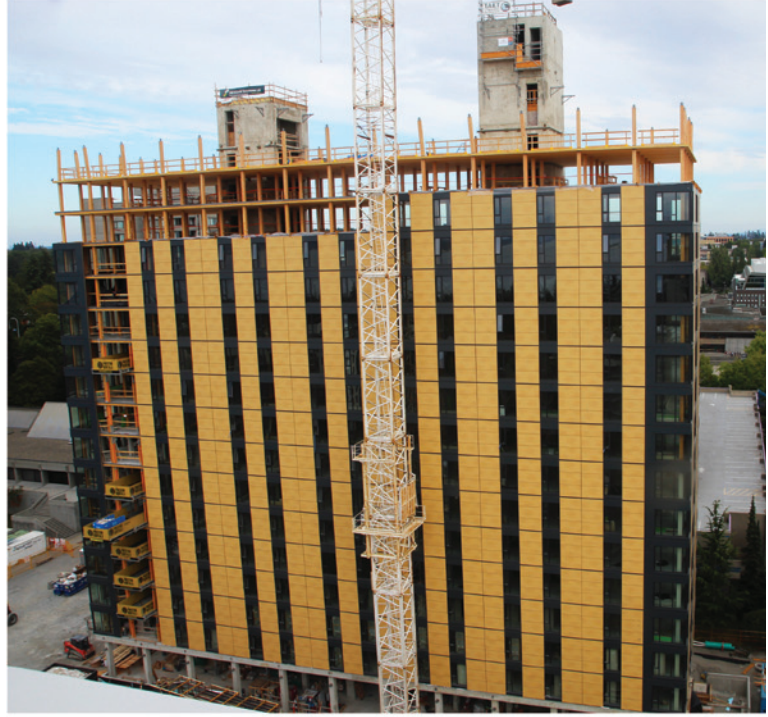
August 2016 concrete construction underway
