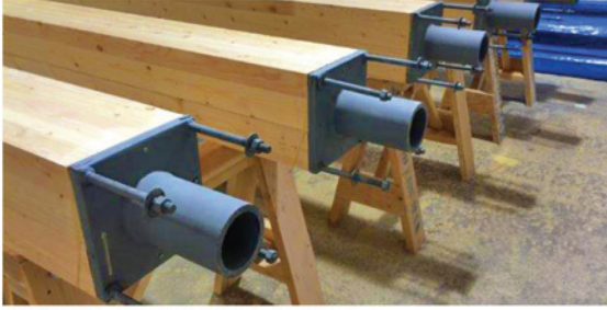
July 2015 glulam columns and steel connectors for mockup
