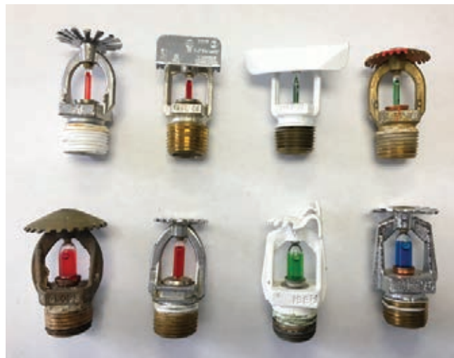
Figure 1. Examples of Standard and Quick Response Bulb Sprinklers
