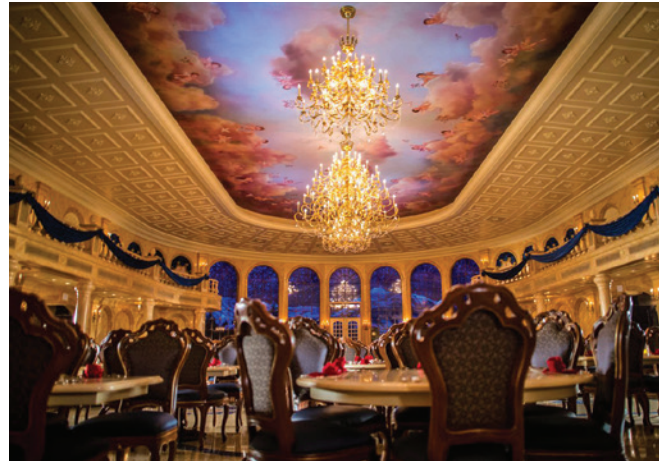
Cloud ceilings that have multiple levels of protection. Sprinklers installed in formed rock work, that mimics a cave, requires multiple trips to install the critical head placement. Finally, as the finished plaster is applied to get the ceiling finish, a final adjustment to check the location so that the sprinkler remains unobstructed for the spray pattern to develop and also that the accumulation of heat will fuse the head in a fire condition.
