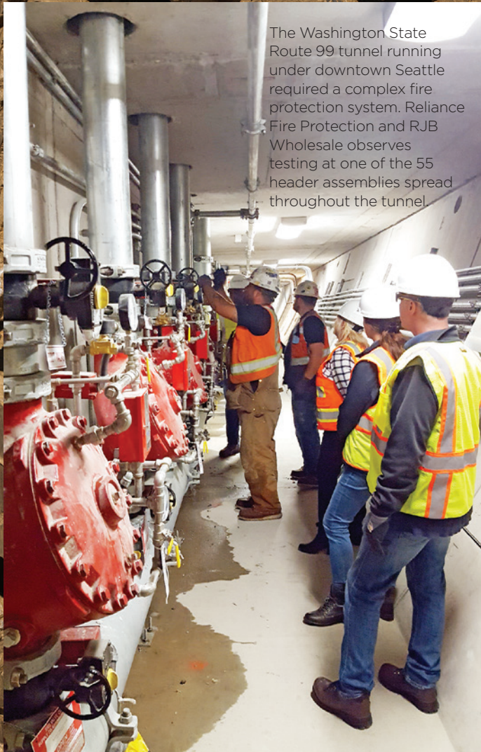
Reliance Fire Protection's Wally Cinkovich and Nancy Hammond, along with RJB Wholesale's Stacie and Nick Beck, observe one of the full flood tests of two of the 208 Roadway Deluge Systems on the newly-constructed Washington State Route 99 tunnel under downtown Seattle.
