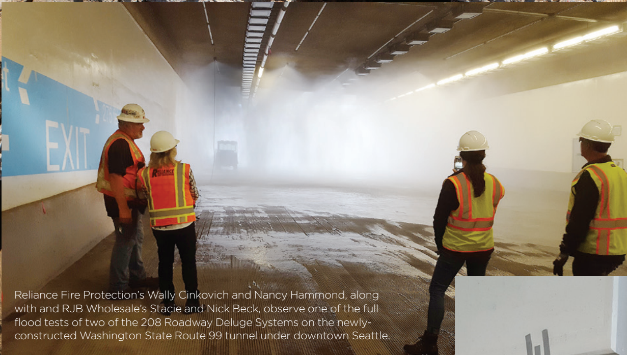
The Washington State Route 99 tunnel running under downtown Seattle required a complex fire protection system. Reliance Fire Protection and RJB Wholesale observes testing at one of the 55 header assemblies spread throughout the tunnel.
