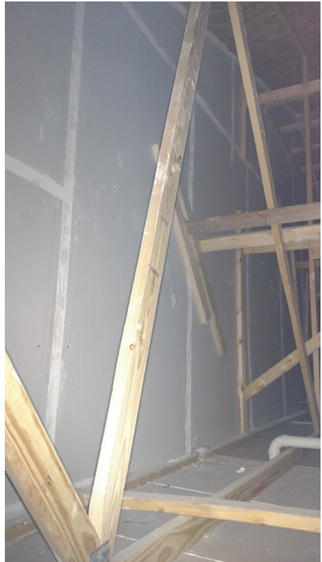
Draftstopping in attic
