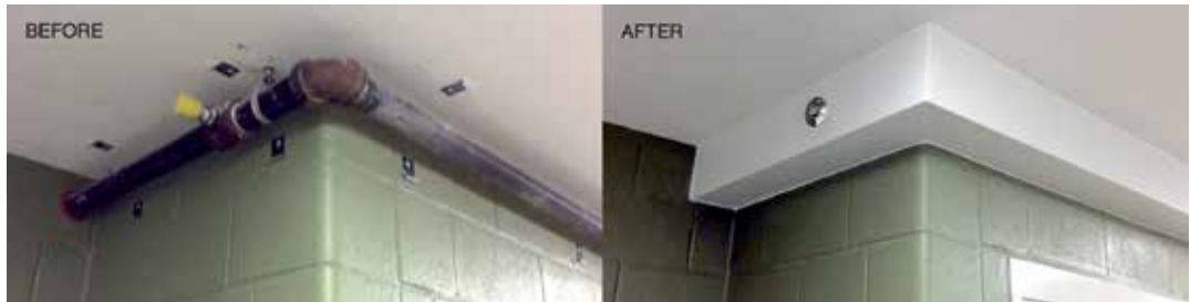
Typical Soffi-Steel® Institutional Application”
