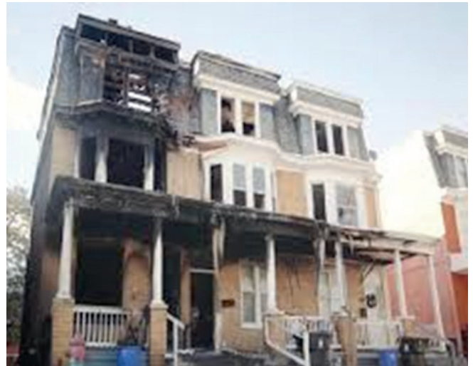
The conditions on Lexington Street after the fire
