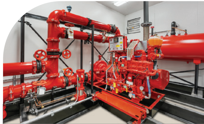
NFPA-20 Diesel Packaged Fire Pump System
