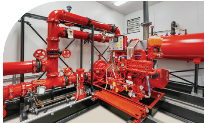
NFPA-20 Diesel Packaged Fire Pump System
