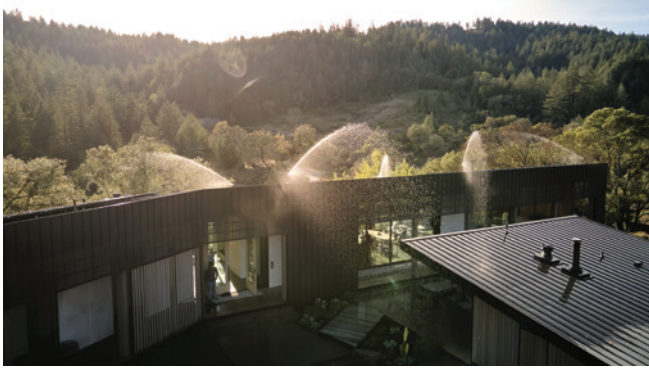
Active roof sprinklers on a new home in Northern California
