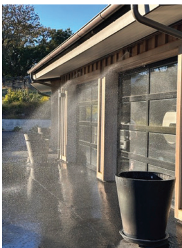
Eave sprays protect the most vulnerable areas of a home
