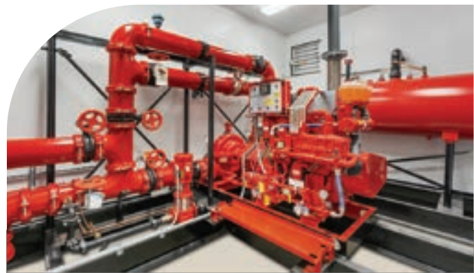
NFPA-20 Diesel Packaged Fire Pump System
