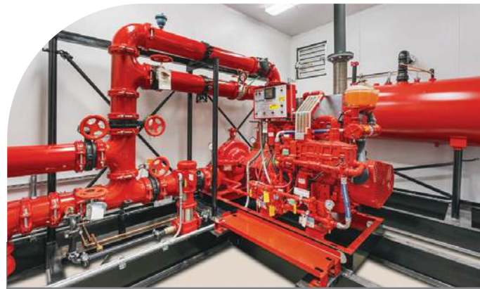
NFPA-20 Diesel Packaged Fire Pump System
