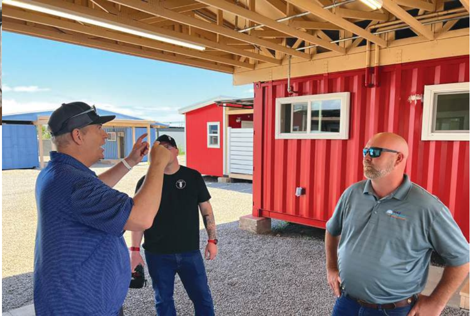
Visiting some of the emergency housing units and checking out some more fire sprinklers.
